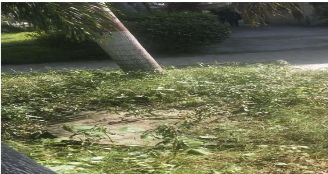
Fig-Rain water harvesting /Ground water Recharge system near History Department
