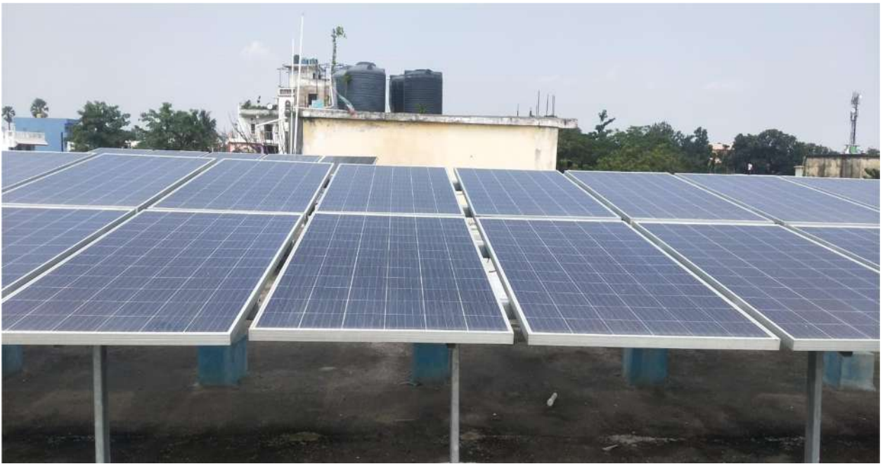
Fig- Solar PV panel system present on the roof of Arts Block
